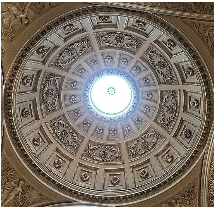
The dome of Gfelkt hahelesgjios
